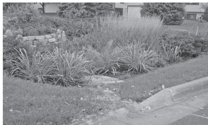
Rain gardens, like this one in Burnsville, are planted in a shallow depression with native vegetation to capture runoff and draw out pollutants. Photo: Barr Engineering
