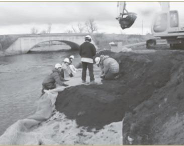
Stabilizing streambanks is one way FMR works to protect the Vermillion River. This 2002 project involved layering willow and dogwood brush between envelopes of soil held by coconut fiber mat.
